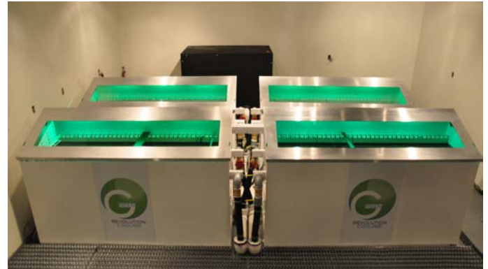
[LEFT and RIGHT]: Perspective views of 100 kW four-rack CARNOTJET™ system installation at Midas Networks
