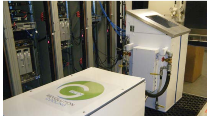
[Left] Dell M1000e blade chassis installed at TACC, [Right] 13U evaluation unit capable of producing 50°C waste water
